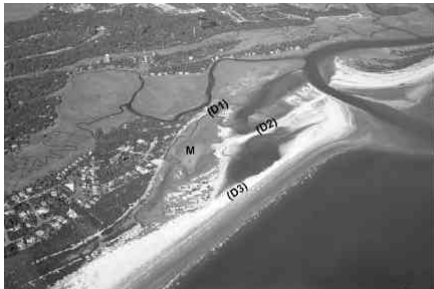
FIGURE 4. Captain Sams Inlet on 16 January 2003. Original floodway before the 1983 relocation is now a 10-hectare salt marsh (M). (D1) Remnant of 1983 closure dike. (D2) 1996 closure dike. (D3) 1998 outer dike.
